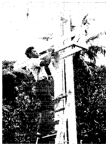
Tom Christian, VR6TC, adjusts a solar-power module on his Pitcairn Island antenna tower. The solar assembly is an alternative power source to the island's costly diesel-powered generator. (photo courtesy Motorola, Inc.)
